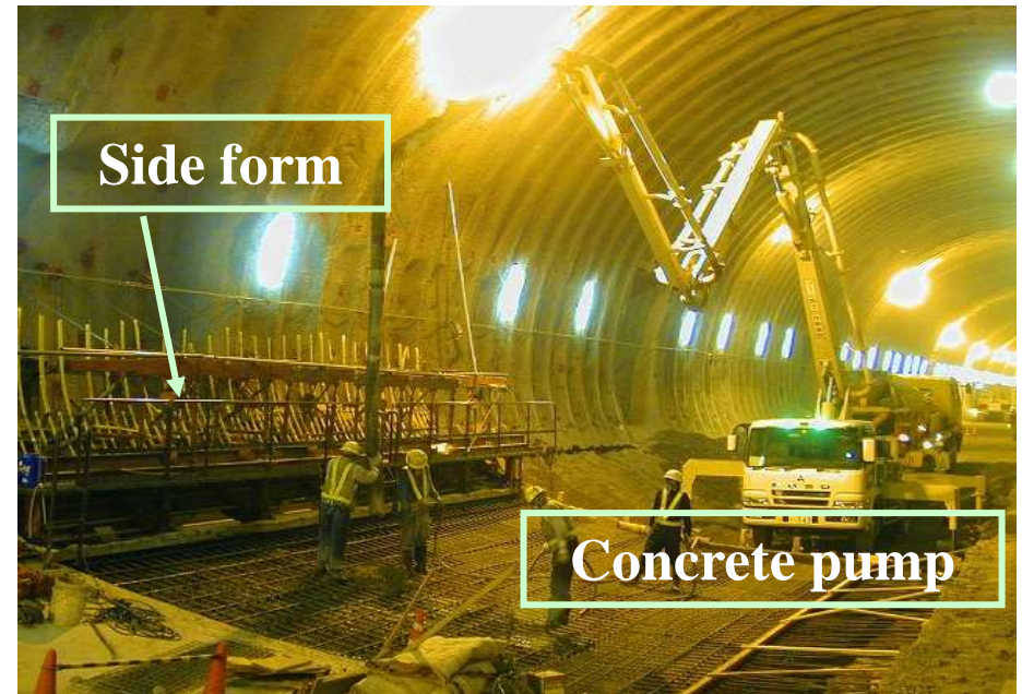
Concrete placing
