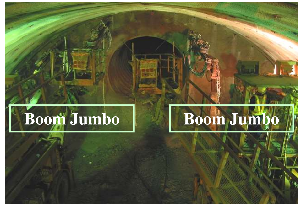
Drilling of charging hole
