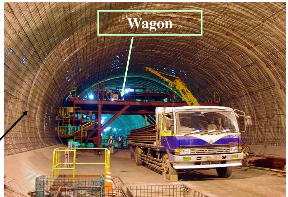
Installation of reinforcement bar
